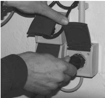
5. Insert cable of pump motor into socket.
